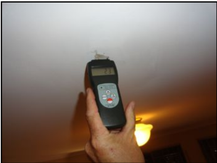
Patched area tested dry
