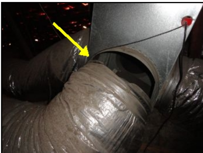
Ducting has come loose from air conditioner splitter box
