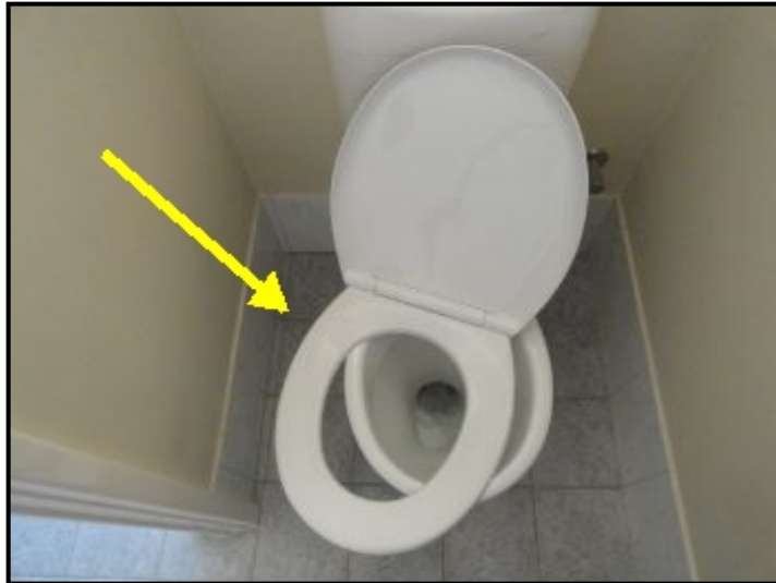
Loose toilet seat noted.
